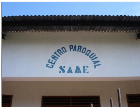
Figure 7.5: Facade name Manufahi, 'Parochial Centre Same', in Portuguese
